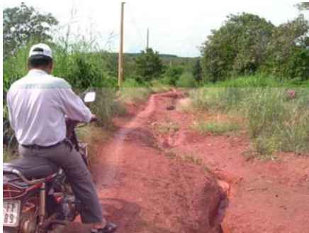
Poor road condition in hamlet 07
